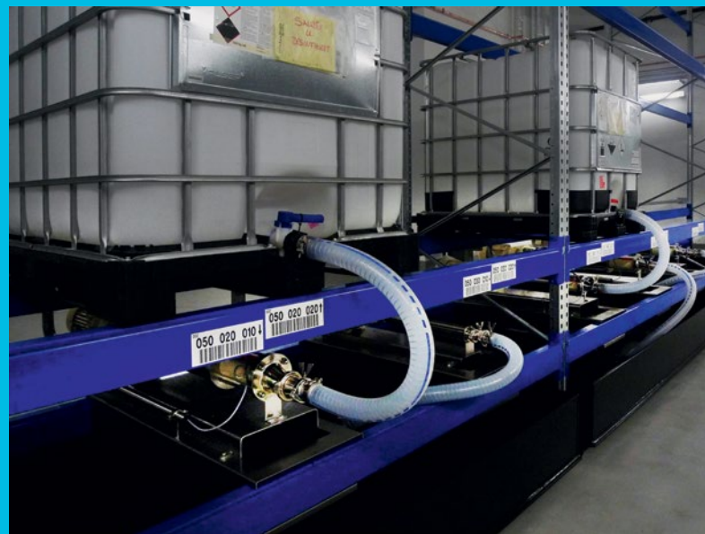
Tank and IBC store with feed pumps
