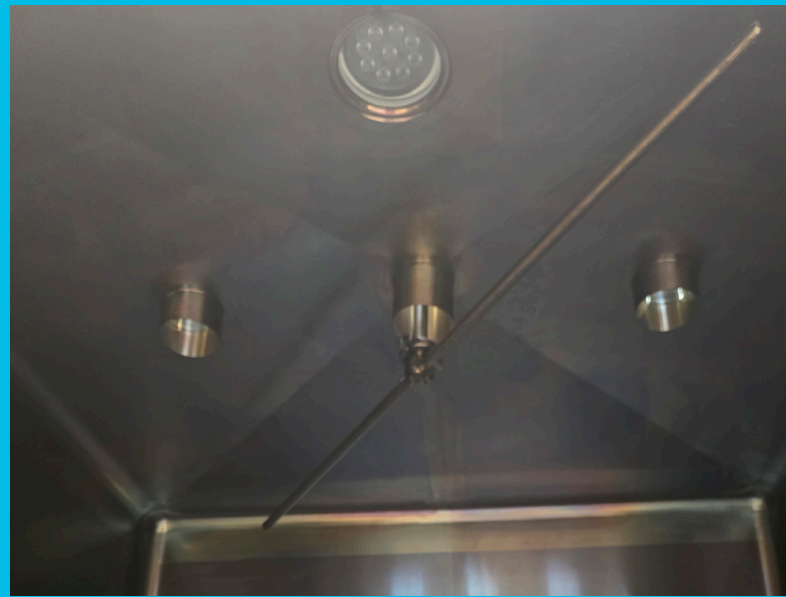
Washing chamber ceiling cleaning
